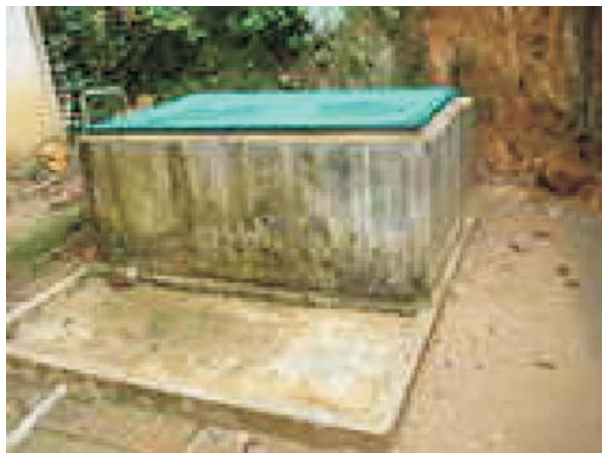
Fig. 2: A photograph of a ground level water storage cement tank covered with a plastic net cover
