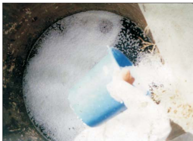
Fig. 1: Application of EPS beads in an abandoned well
