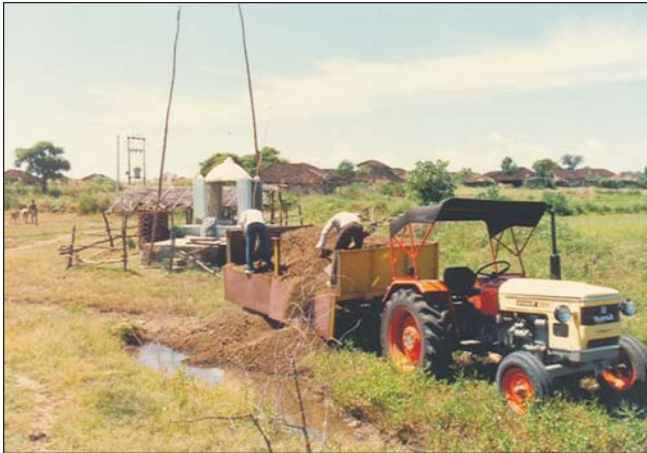
Fig. 2: Source reduction by filling earth
