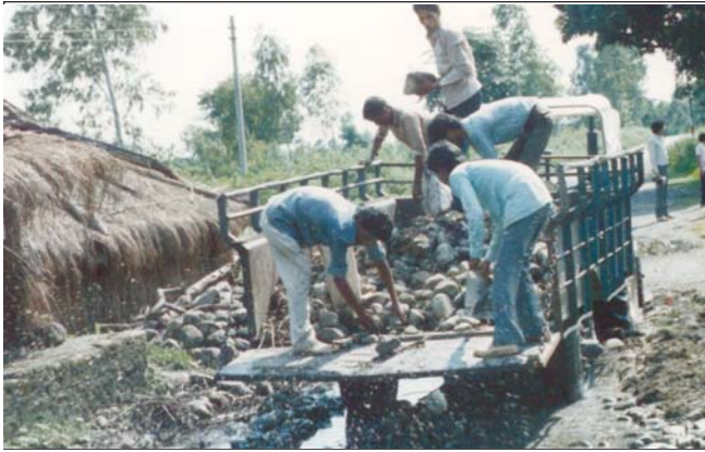
Fig. 2: Filling-up of mosquito breeding habitats with earth and stones
