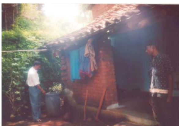
Fig. 3.1.12: Kuchcha houses in Madhya Pradesh
