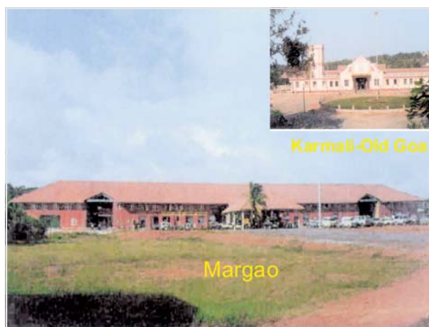
Fig. 115: Konkkan Railways Station at Margao and Karmali-Old Goa (Inset). With the timely intervention of NIMR, the design of station building was changed by the Konkkan Railway Corporation and sloping roofs were provided to prevent water stagnations on station terrace during heavy monsoons experienced in the Konkkan Region
