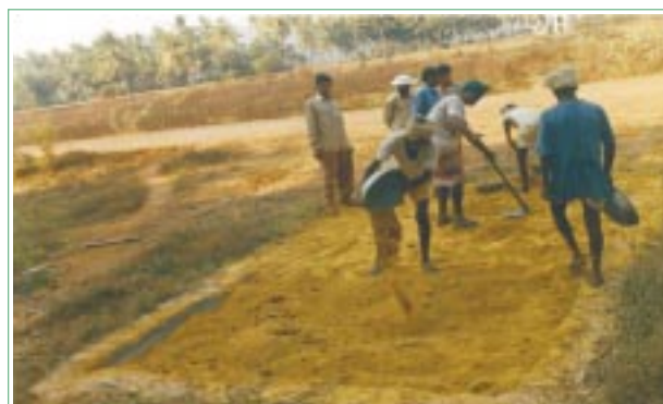
Tank being leveled with earth
