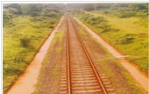
Drains on sides of track
