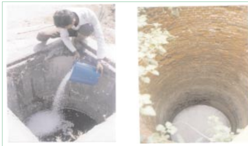
Application of EPS beads in unused cement tanks and wells
